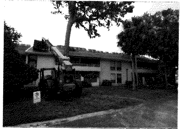
Condominium Building Roof Project in Progress
