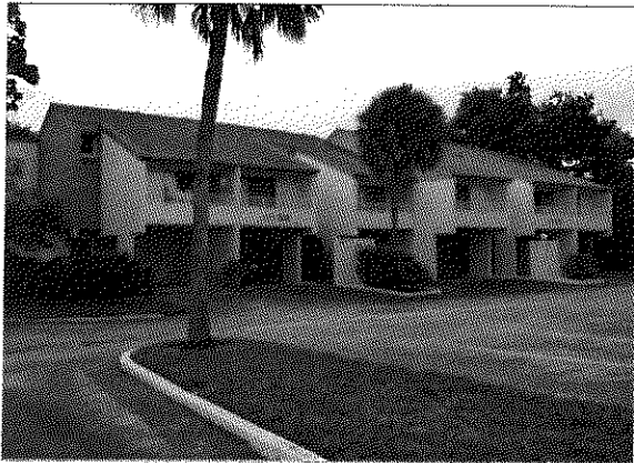
Condominium Building Front View
