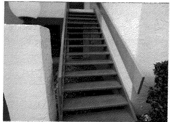
Condominium Building Stairway
