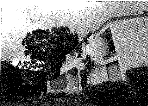
Condominium Building Rear View
