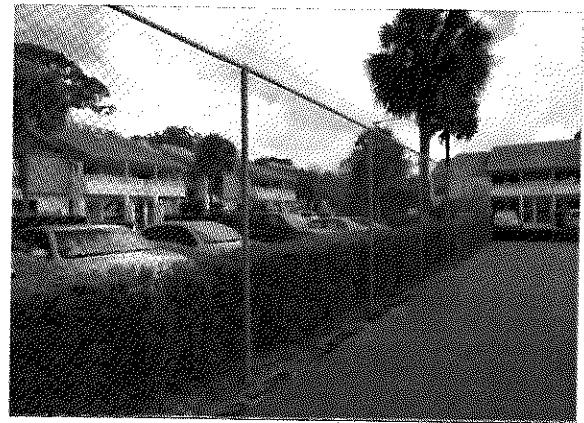
Tennis Court Fencing
